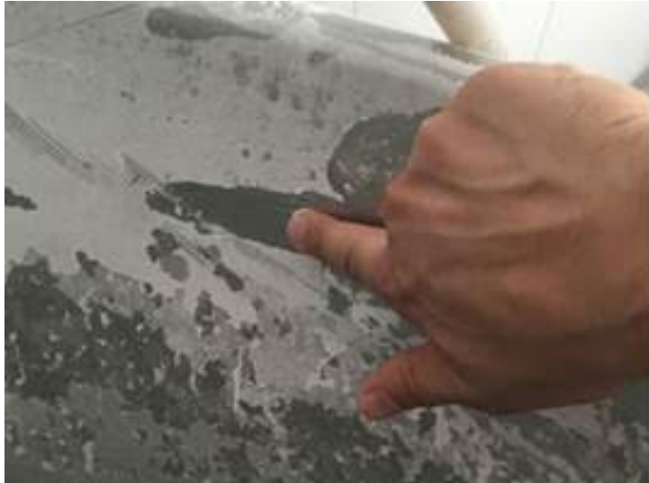
Figure 5 – Surface deposit of calcite powders without inter-particle cohesion
